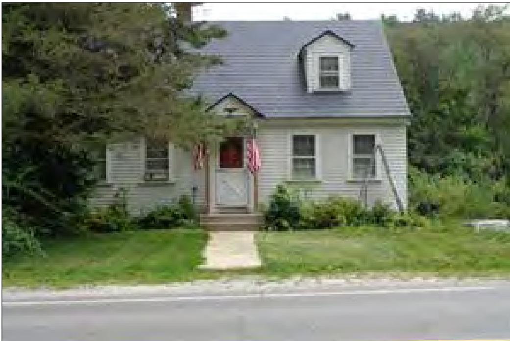
Photo 8 – 49 Mont Vernon Road (Tax Map 19 / Lot 4, Est Construction 1950)
