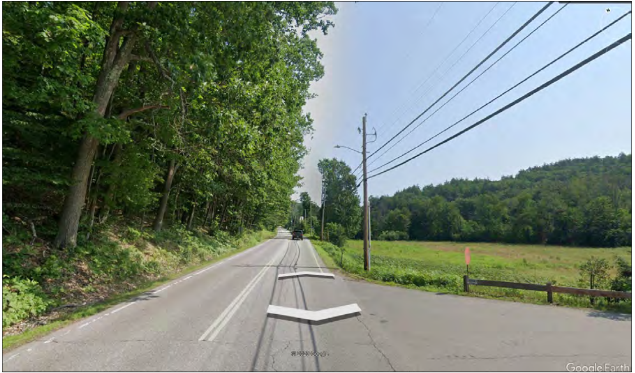
Photo 1 – Mont Vernon Road Looking North – Proposed Fire Station Site Pictured to the Right
