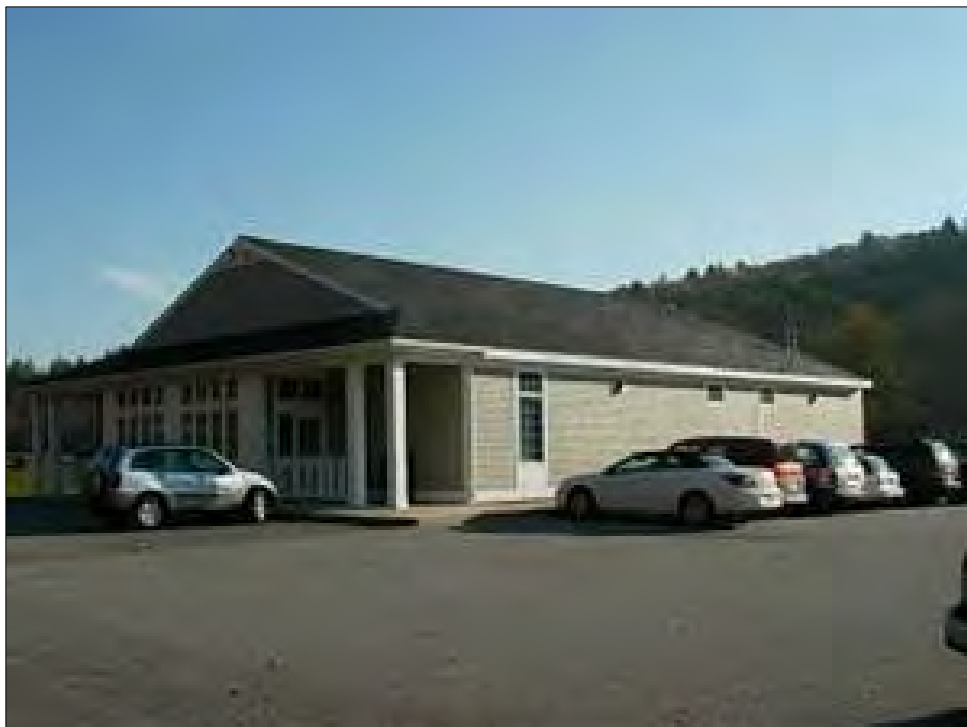
Photo 4 – 71 Mont Vernon Road (Tax Map 8 / Lot 110-1, Est Construction 1997)
