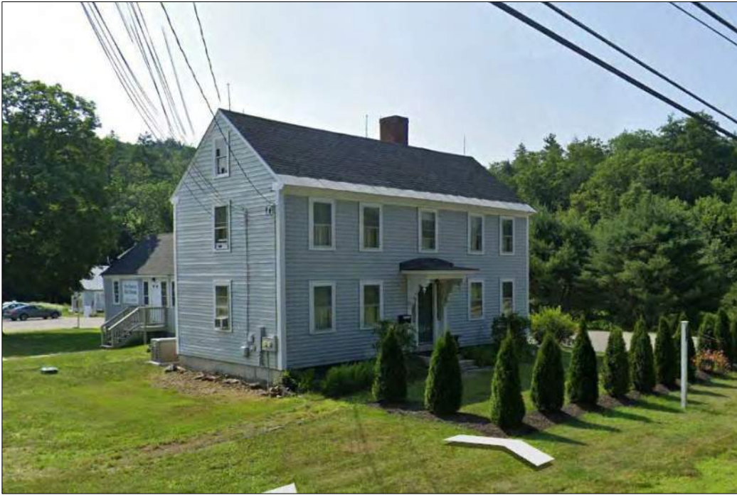
Photo 5 – 71 Mont Vernon Road (Tax Map 8 / Lot 110, Est Construction 1900)
