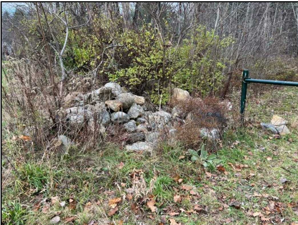
Plate 5. View North-Northeast of the Stone Wall Where It Was Broken to Accommodate the Gate
