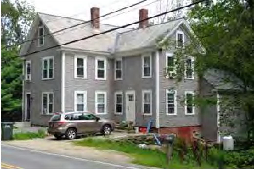
Photo 9 – 45 Mont Vernon Road (Tax Map 19 / Lot 5, Est Construction 1900)
