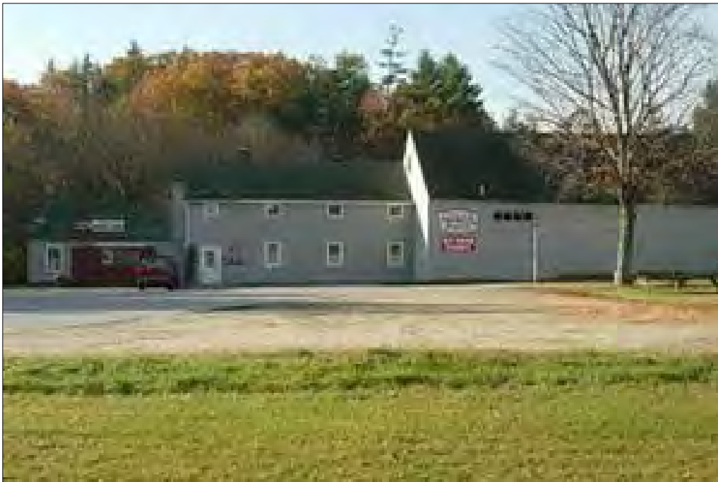
Photo 6 – 81 Mont Vernon Road (Tax Map 8 / Lot 110, Est Construction 1900)
